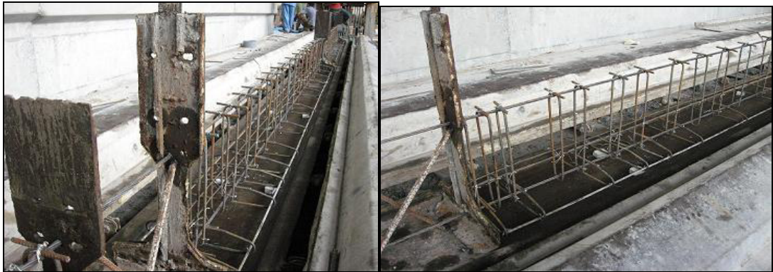
Figure 3. Prestressing steel and shear reinforcement locations
